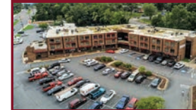
1835 University Boulevard East Hyattsville, MD 20783 524 & 850 SF Office Space
